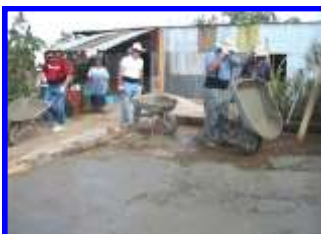
Pisos's, Latrines, Chicken Coops, Mexico
